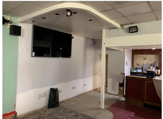
At the start of the main refurbishment, there was a lot of unseen work that had to take place including lifting and removing bags of asbestos floor tiles and repairing the old concrete floor underneath. We then had a damp proof membrane fitted to help insulate the Club for the future. Members have also fitted a new floor to the meeting room to finish that part of the project.
